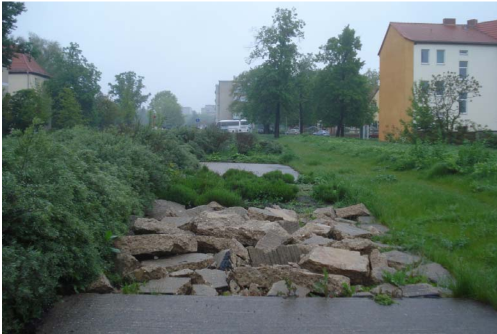
Figure 7.2. Road deconstruction in Dessau
