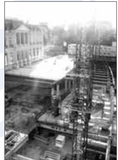
Bright prospects for the new conference centre as work continues apace.
