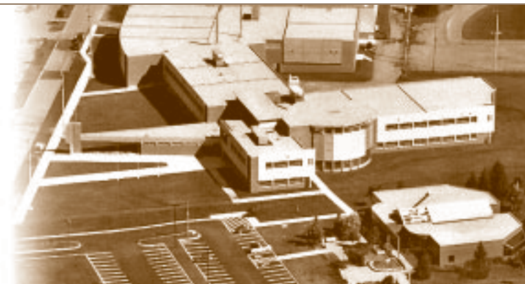
The Odysée secondary school in Val-Bélair, Quebec, shares its sports facilities with the city in exchange for use of the municipal library (lower right).
