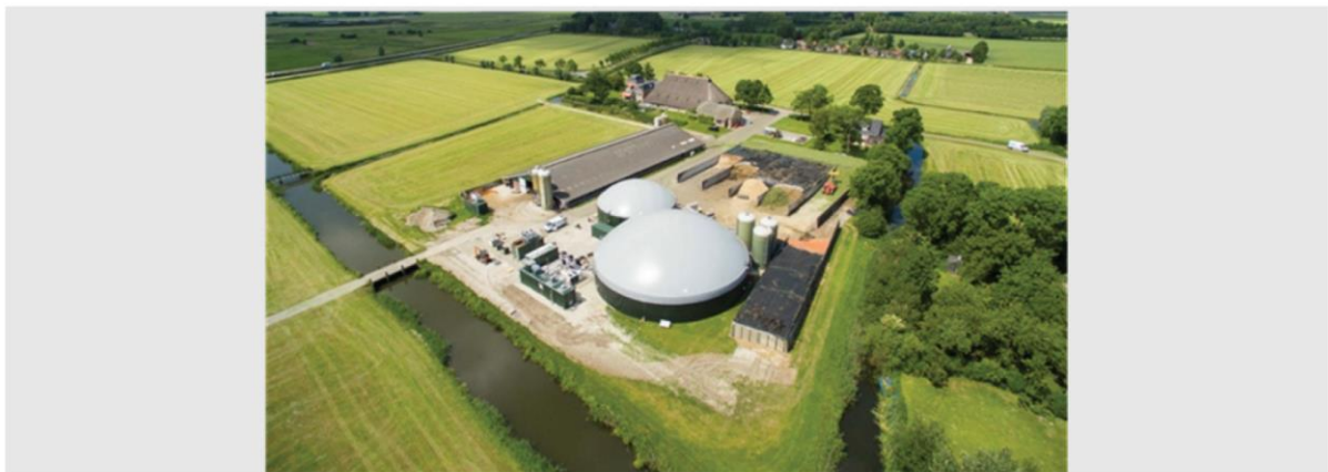
Figure 4.3. Farm-scale anaerobic digester, Jelsum, Netherlands
