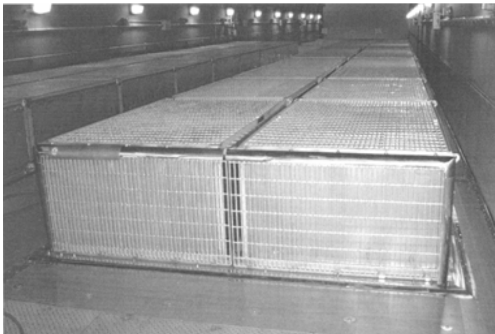
Figure 8. Darlington NGS Finned Strainer
