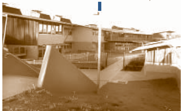
Camden High School, with "solar chimneys"
