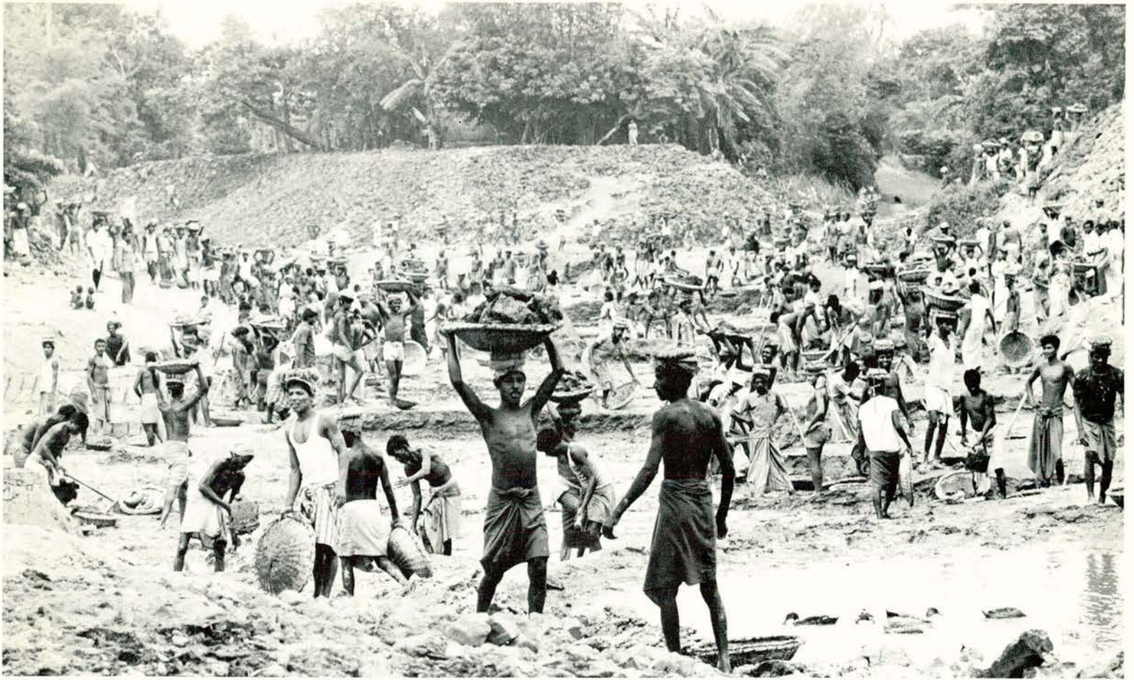
Desilting the Mohadevpur River in Bangladesh—a World Food Programme project—to increase food production: workers are paid in kind.
