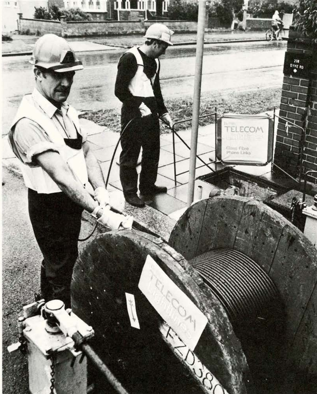
Optical fibre cables are expanding network capacity but require large-scale investment.
