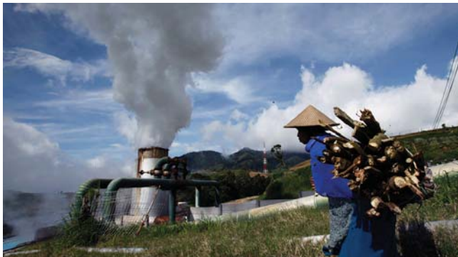
Geothermal plant in Indonesia
