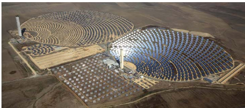
Figure 2: View of Abengoa's Plataforma Solar Sanlucar La Mayor near Seville, Spain, with the 11 MW PS10 and construction of the 20 MW PS20 (Abengoa Solar)
