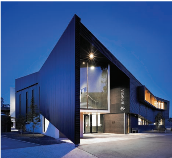
Figure 7. Entry to one of the seven houses.
