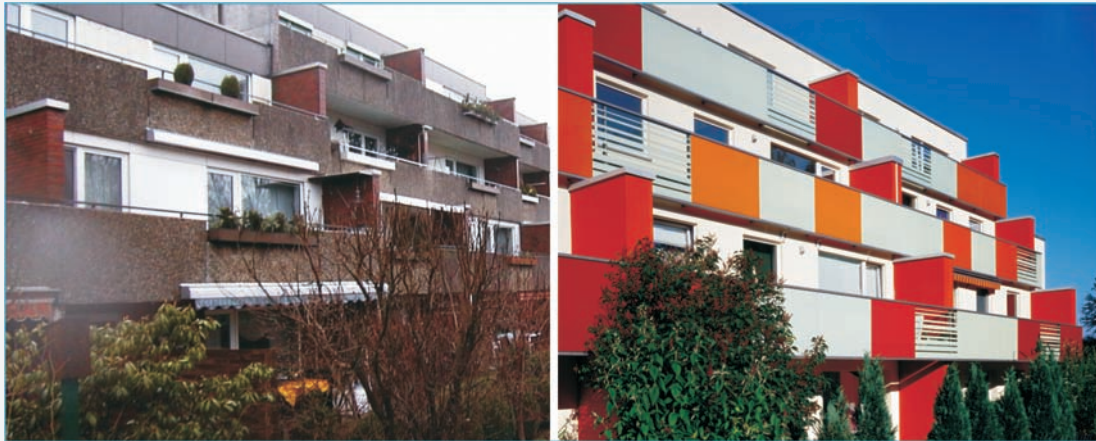
Figure 3.11 Wall retrofit for energy efficiency with EIFS
