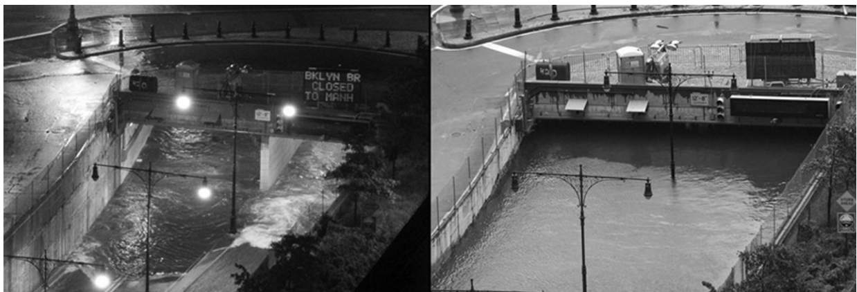
Figure 2.15. Flooded NYC tunnel due to Hurricane Sandy storm surge and infiltration
