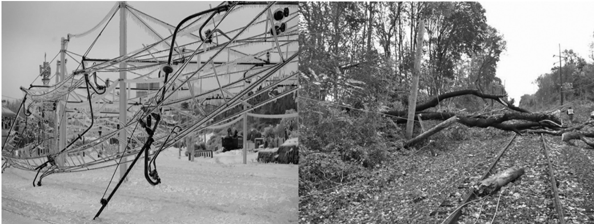
Figure 2.19. Ice damage to rail overhead structures and storm-fall on rail tracks
