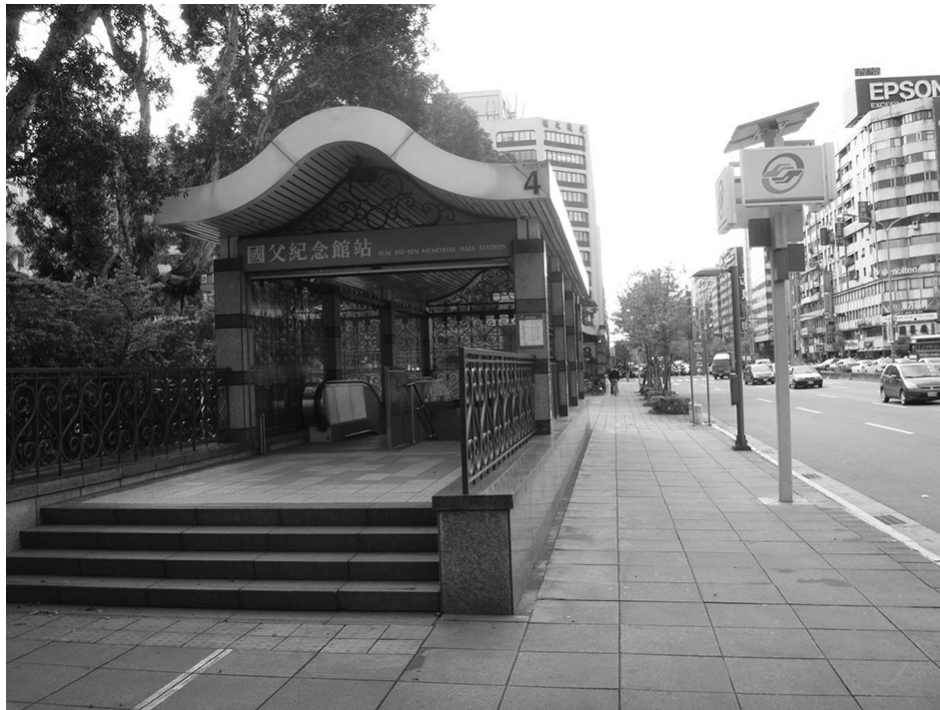
Figure 2.20. Raised subway entrance to prevent pluvial tunnel flooding, Sun Yat-Sen Memorial Station, Taipei Metro, Taipei
